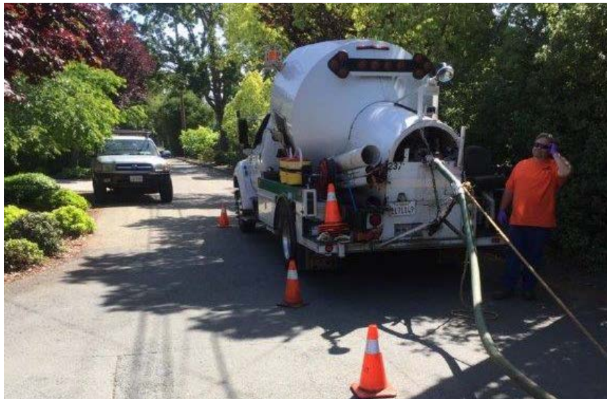
Figure 4.2 Central San Rodder Truck
