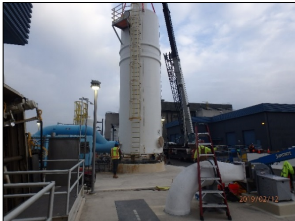
Rehabilitating the odor control tower under the Mechanical and Concrete Project
