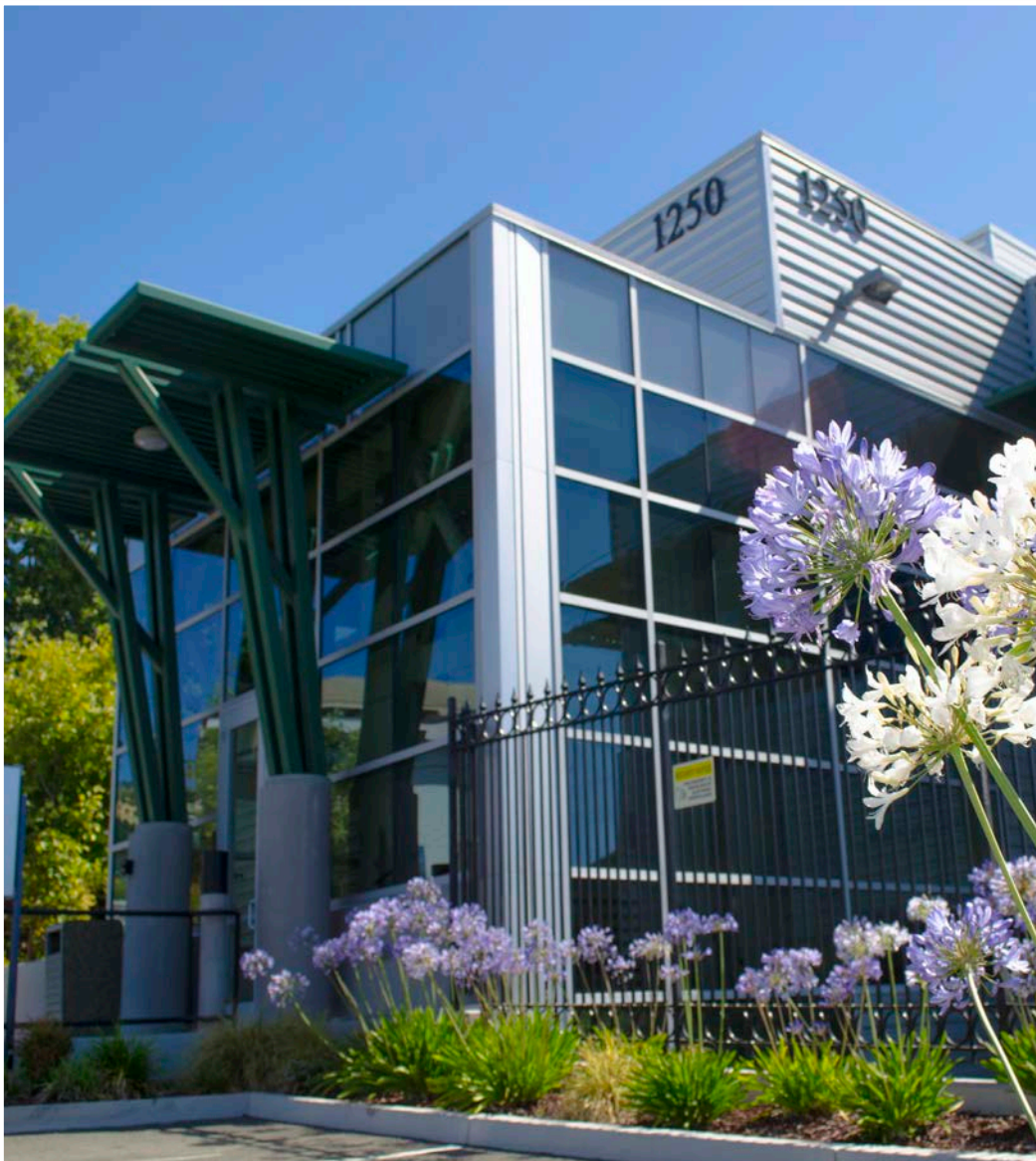
The bold design of the Collection Systems Operations building.
