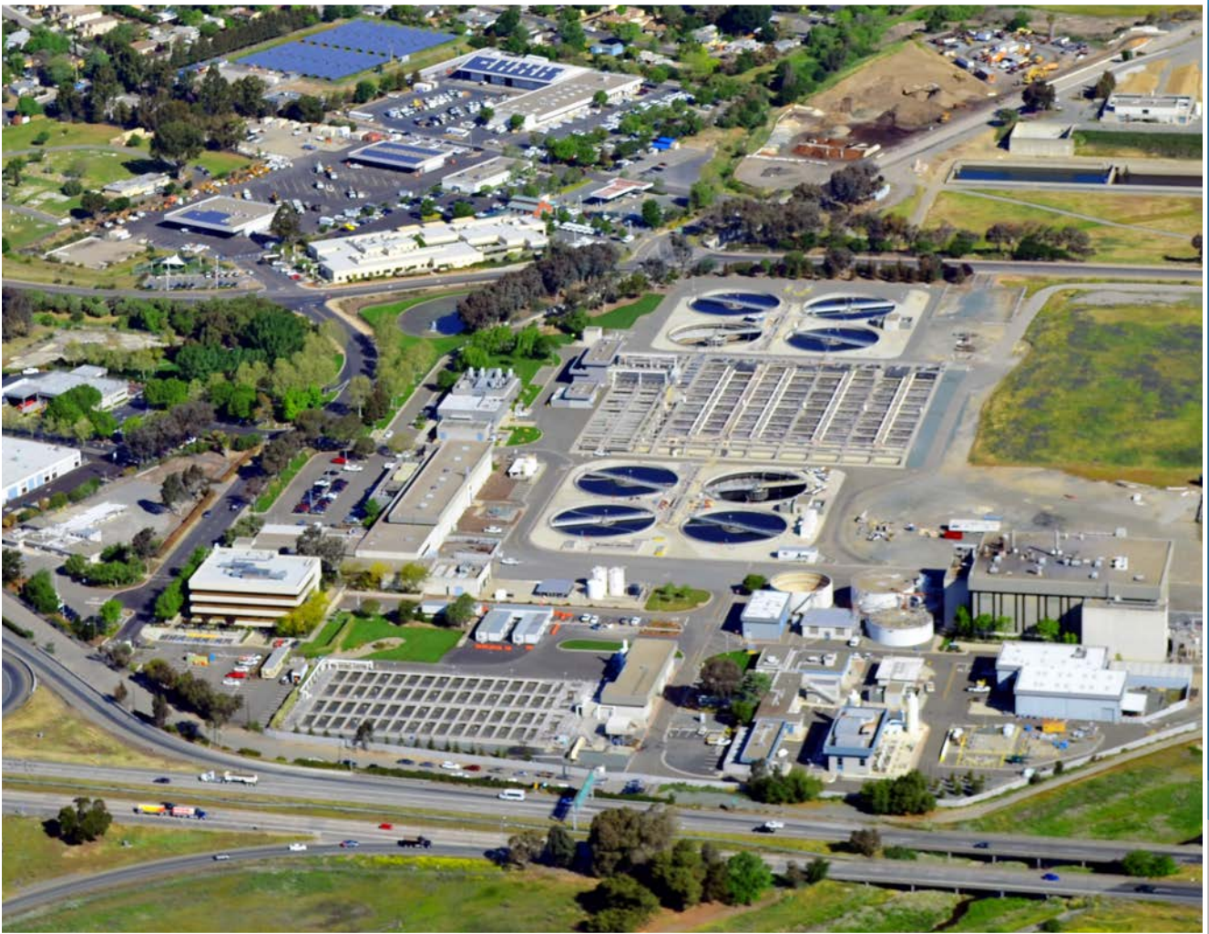
Aerial of the Martinez Treatment Plant, April, 2013.
