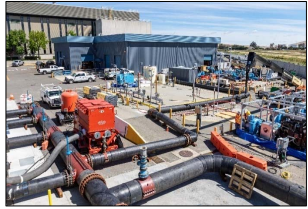
Rehabilitating the odor control tower and temporary bypassing under the Mechanical and Concrete Renovations Project
