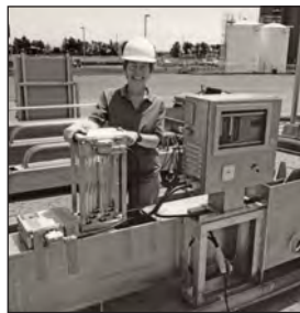
Pilot testing ultraviolet light disinfection
